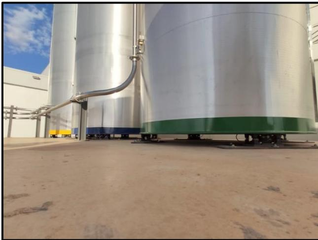
Fig. 1 - Skirted silos used for storing Polymer granules.
